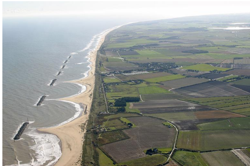
Figure 2.4: Sea Palling Offshore Breakwaters
