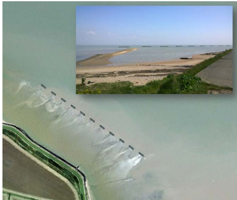
Figure 2.6: Beached barges to protect against coast erosion at Bradwell-on-Sea
